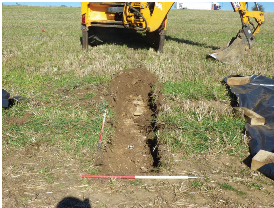
Soakaway 28, general view, looking north
